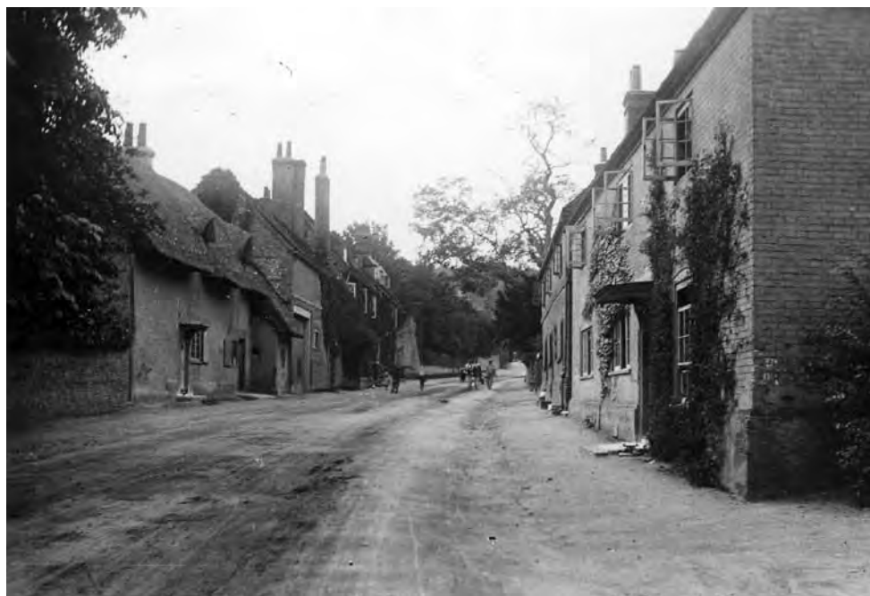
Streatley High Street in the 1920s showing numbers 6-8 on the right [GSLHS collection]
