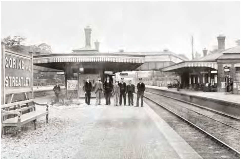
Goring and Streatley Station in the late 1890s, soon after widening [Didcot Railway Centre]
