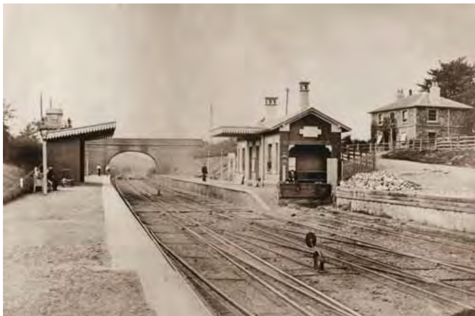
Goring Station with mixed gauge track [GGLHS collection]
